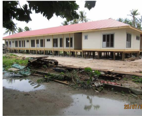
Google Earth image Fenua Fala hospital (left), the new Fenua Fala hospital near completion.
